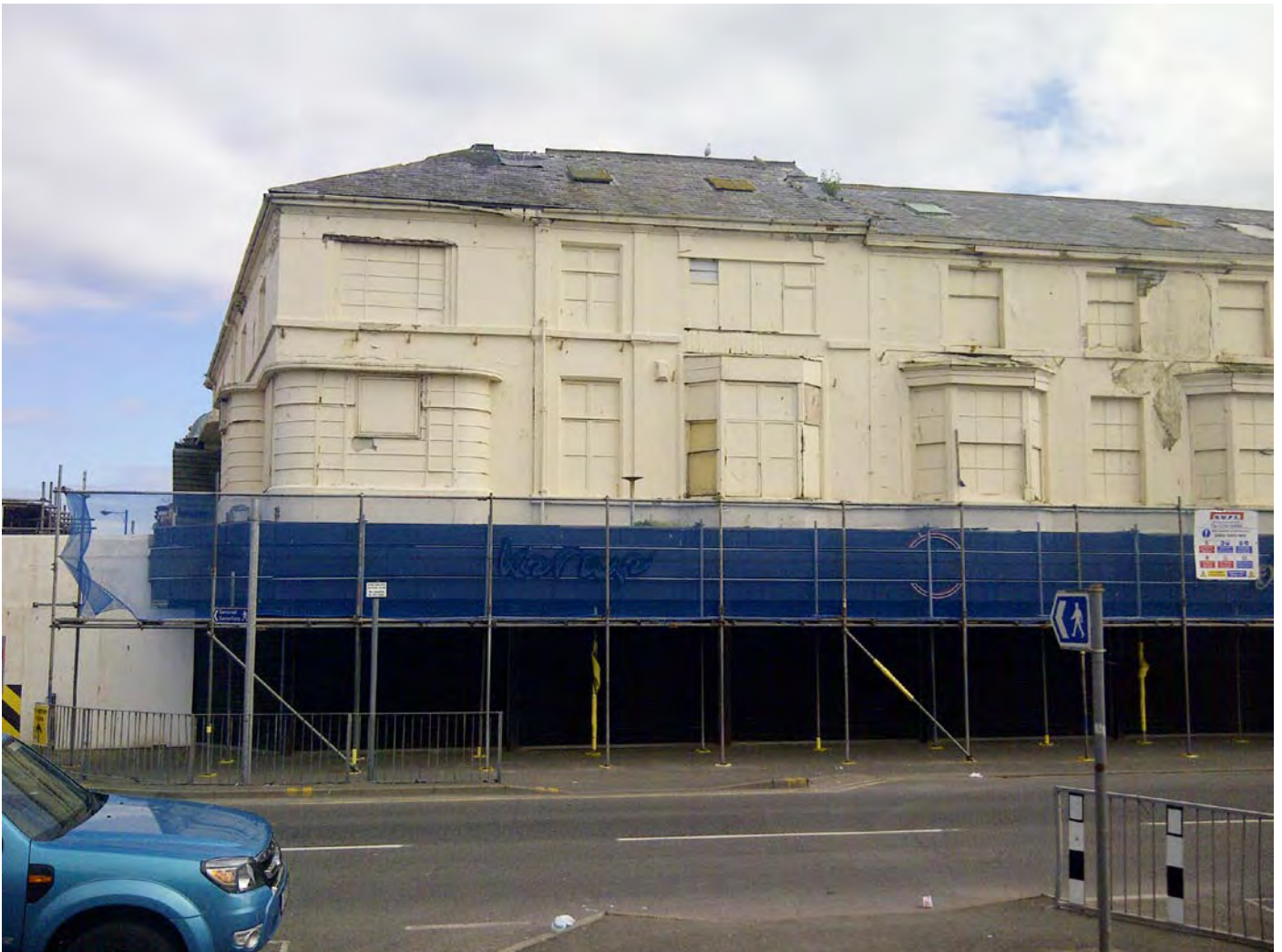
West Parade/Water Street Development site
