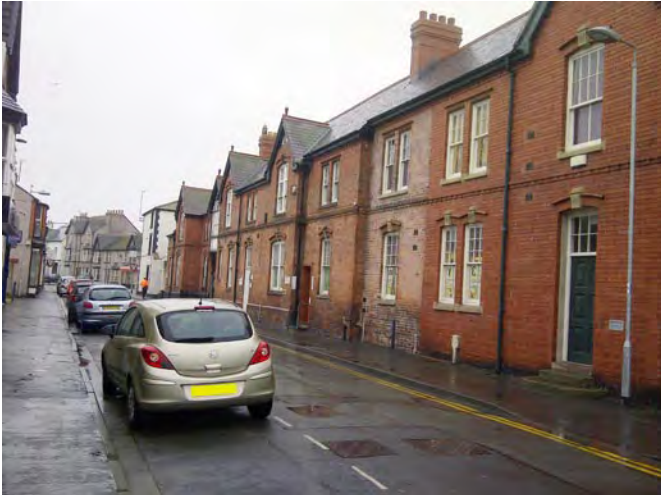
Two storey red brick properties Bedford Street
