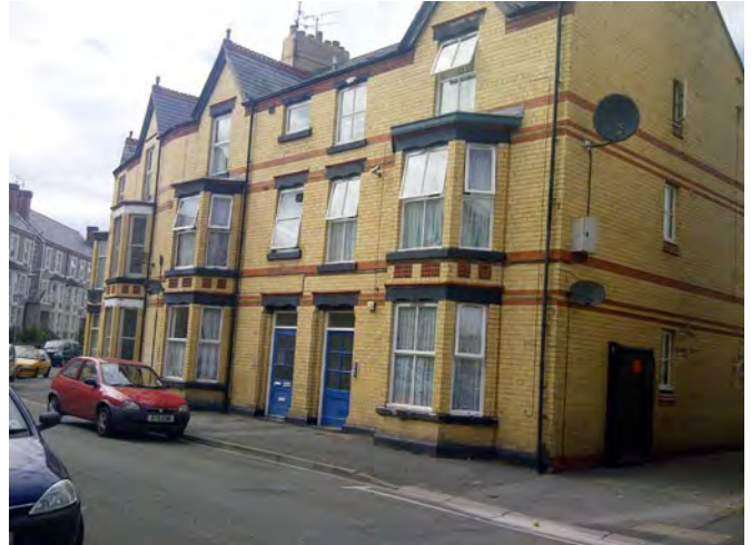
Yellow brick housing, terracotta panel and cill bands, Conservation Area Edward Henry Street east
