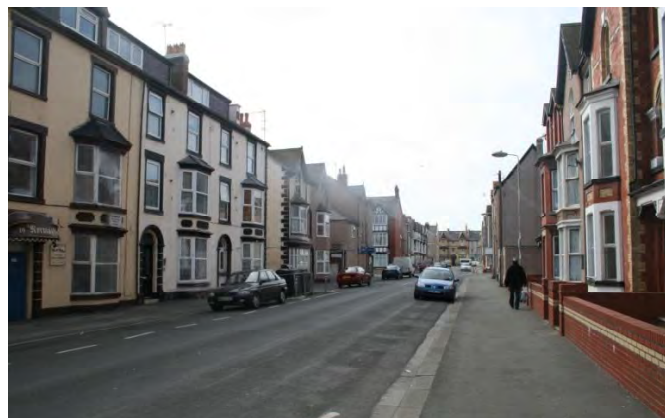
Aquarium Street. West Rhyl. Existing building form, line and massing
