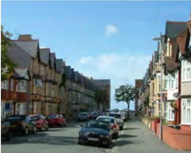
River Street traditional 2 and 3 storey bay fronted properties
