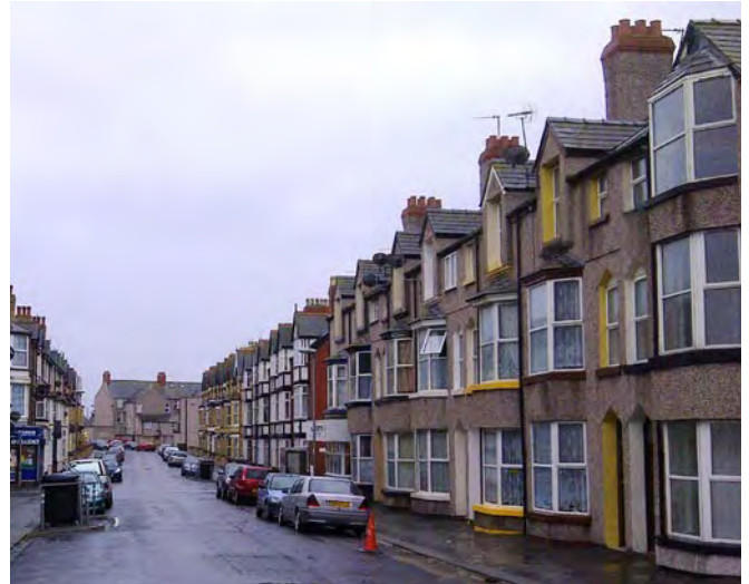
John Street 3 storey bay fronted properties
