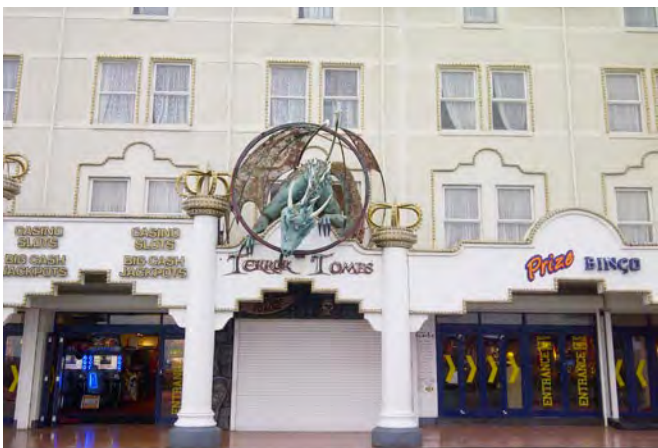
Four storey properties West Parade with commercial ground floor uses
